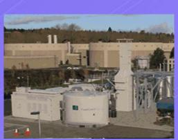
Fuel Cells turn natural gas into electricity
