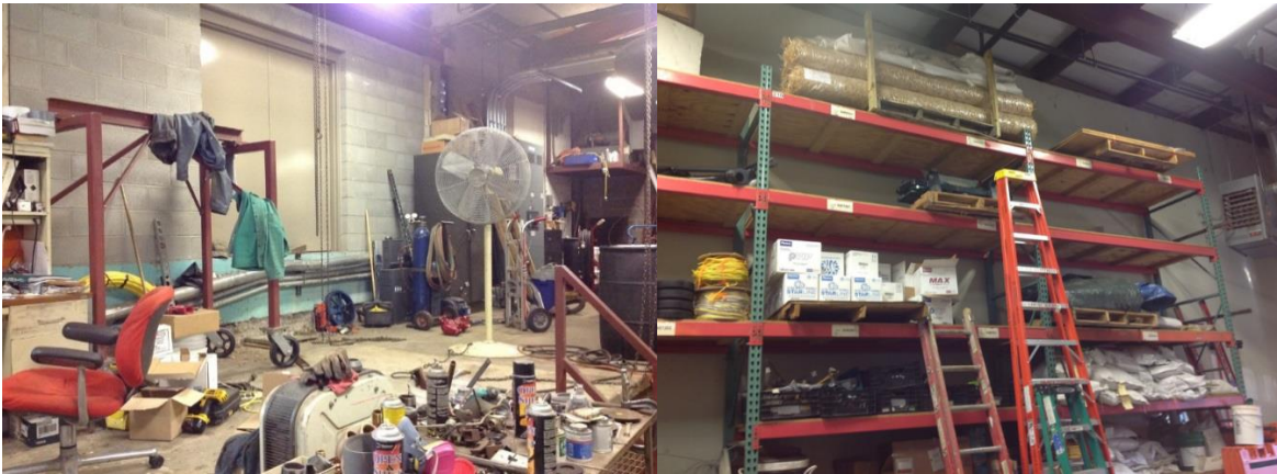
Figure 24: Boiler Room (left) and Physical Plant Warehouse (right)
