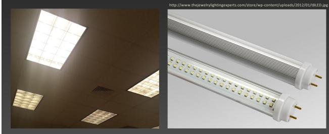
SB 120 (Current) 3 bulbs per fixture 30 watts/bulb 90 Watts De-lamp and replace with LED's 2 bulbs per fixture 18 watts/bulb **36 Watts**   $http://image.dhgate.com/albu\_485628563\_00-1.0x0/t8-1-2m-double-lighting-fixture-brackets.jpg$
