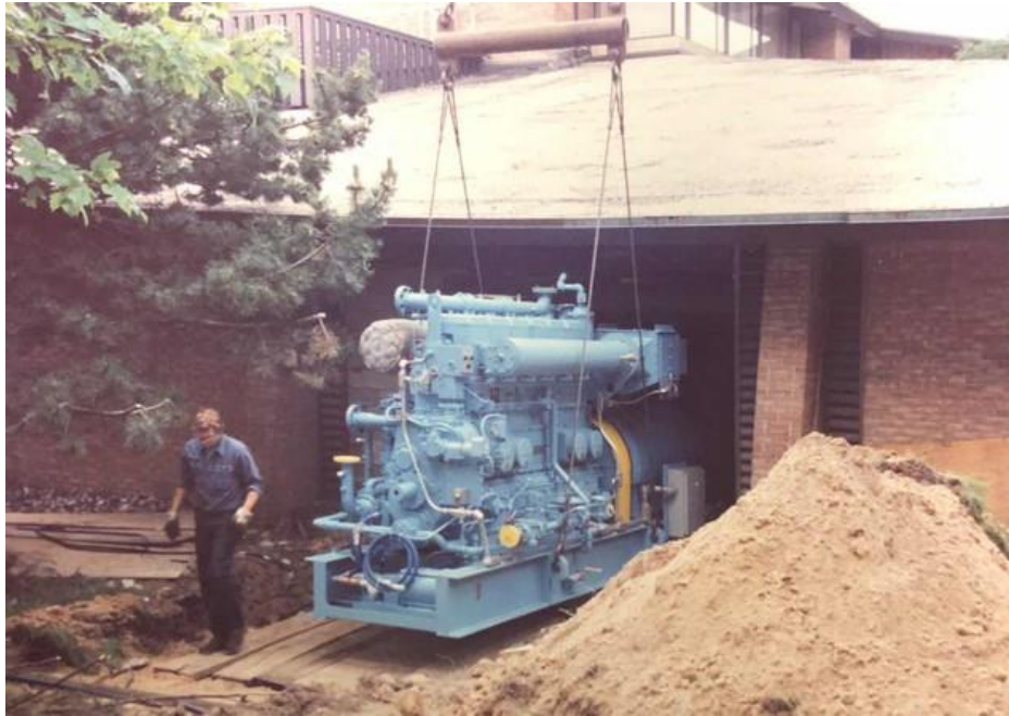
Figure 2.1: Installation of Previous Co-gen (1990)
