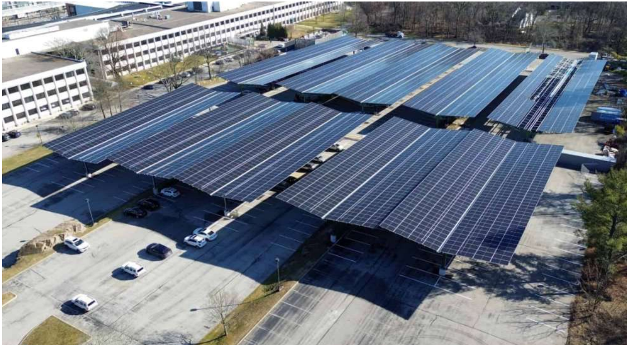
Figure 26. Y-Frame Solar Car Park made by Solar Mounts LLC, like what would be proposed at Calvin.
