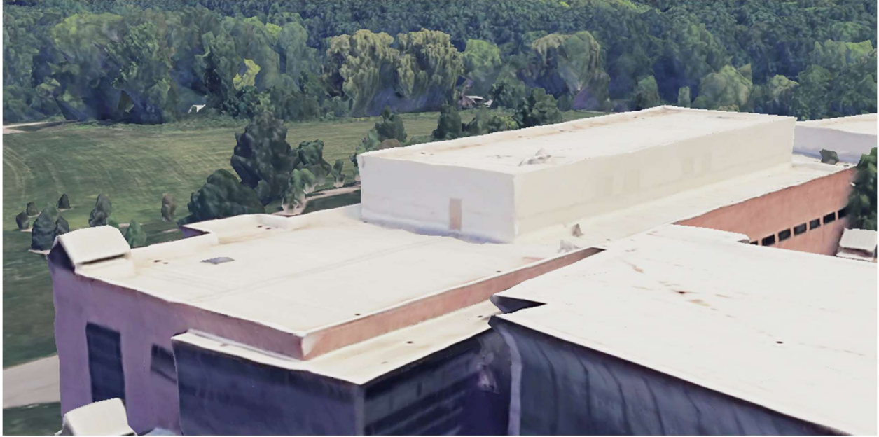
Figure 6. Side View of Communications Building Roof.
