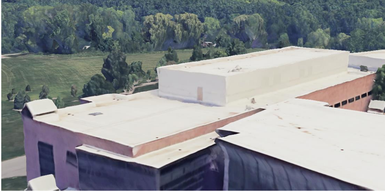
Figure 6. Side View of Communications Building Roof.
