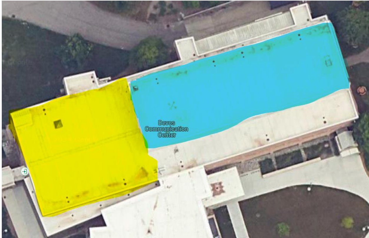
Figure 5. Roof Sections of Devos Communication Center.
